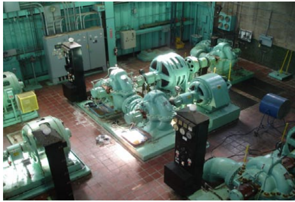
Public water pump room – note blue fan blowing on rings to reduce potential of brush hydroplaning
