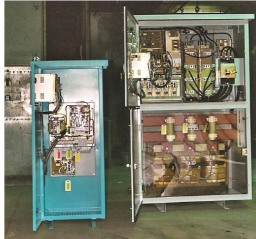
Left: Off-shaft brushless motor excitation system Right: Brush or slip ring motor excitation system
