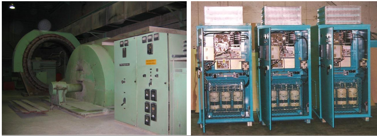
6000 Hp, 1950's vintage, paper mill chipper motor excitation retro-fitted with solid state excitation system
